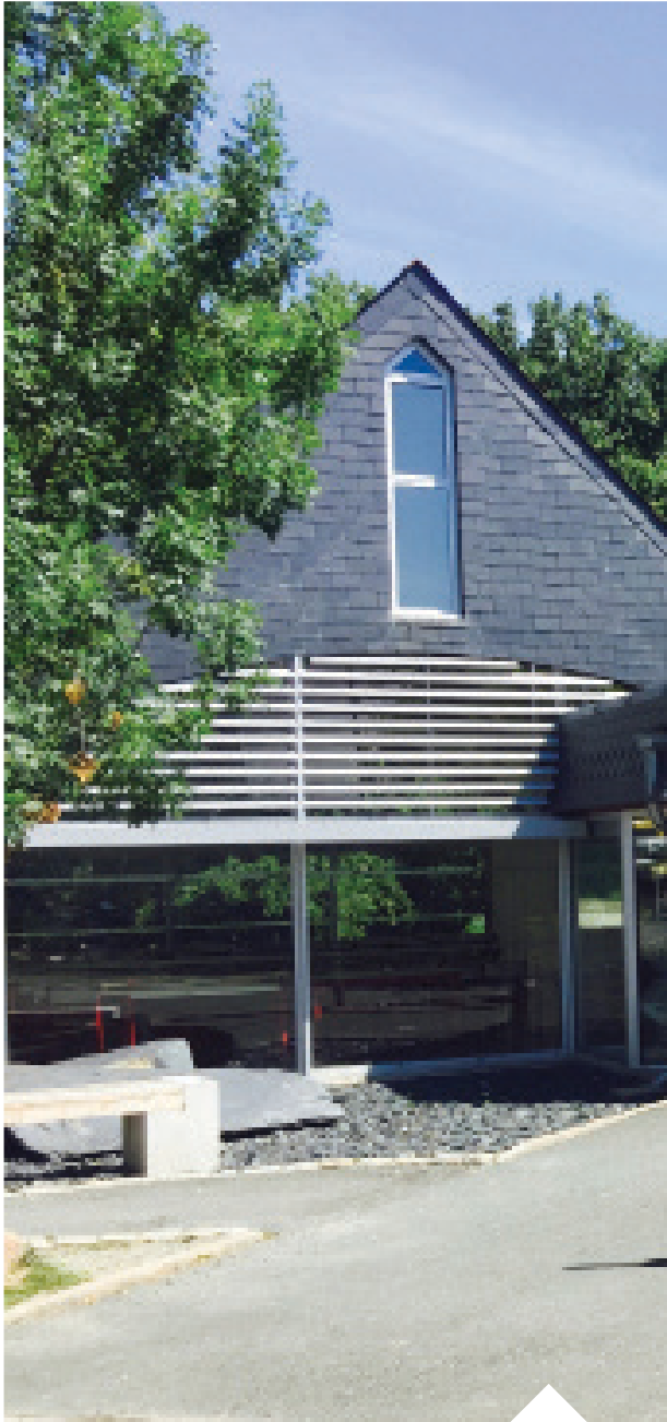
Restaurant, LA POUËZE (49) Architect: SARL Terrien Architectes | Installation: Menuiserie Menard
