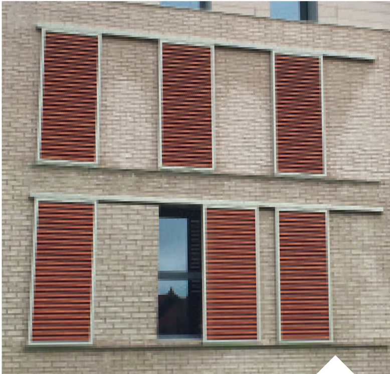
Sofim, CYSOING (59) Architect: Agence HAWA | Installation: Secoferm
