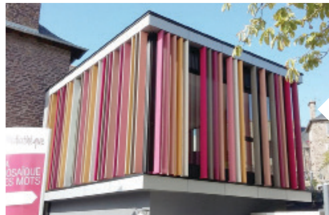
Multimedia Library, IFFENDIC (35) Architect: Quator | Installation: Ser.AL.Fer
