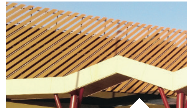
Carrefour, VILLIERS-EN-BIÈRE (77) Architect: ASE PRODUCT Architectes | Installation: Galopin
