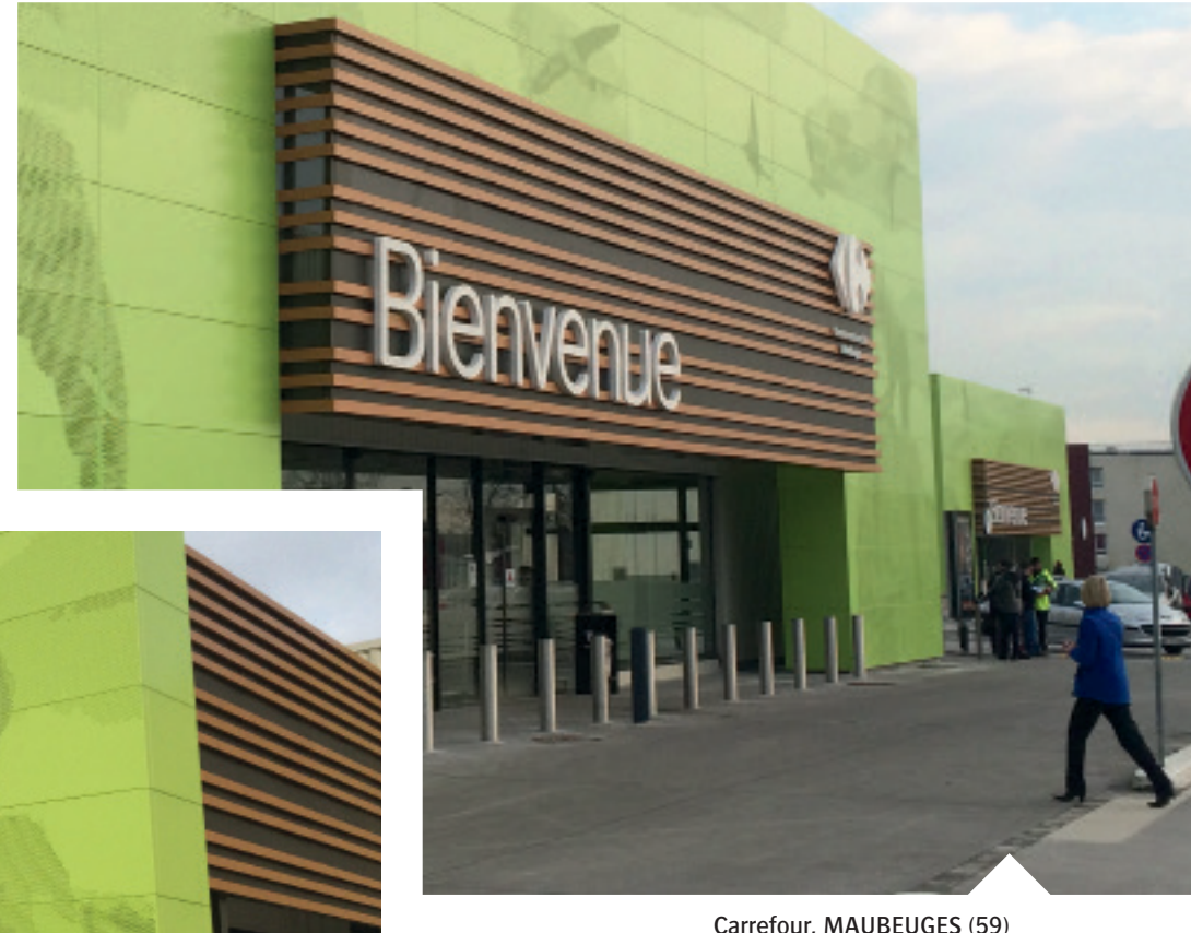
Carrefour, MAUBEUGES (59) Architect: Guerin & Pedroza | Installation: Isobac Acier
