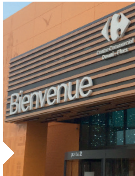
Carrefour, DOUAI (59) Architect: ASE PRODUCT Architectes | Installation: Isobac Acier
