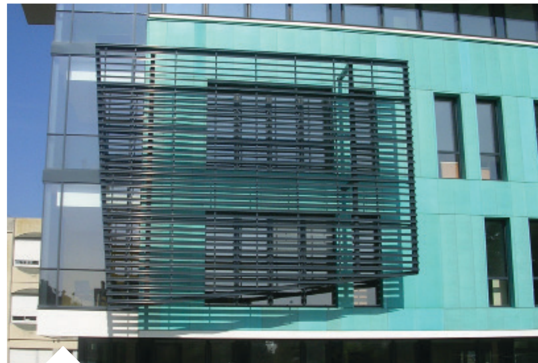
ESA, ANGERS (49) Architect: ESA Cabinet Rolland | Installation: Ets Brault
