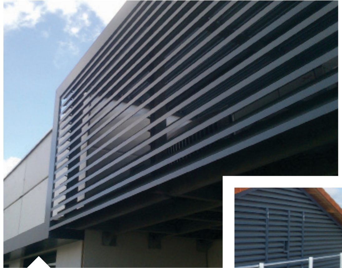
Ephad, CORON (49) Architect: AD Quation & Arcature | Installation: Caillaud bois
