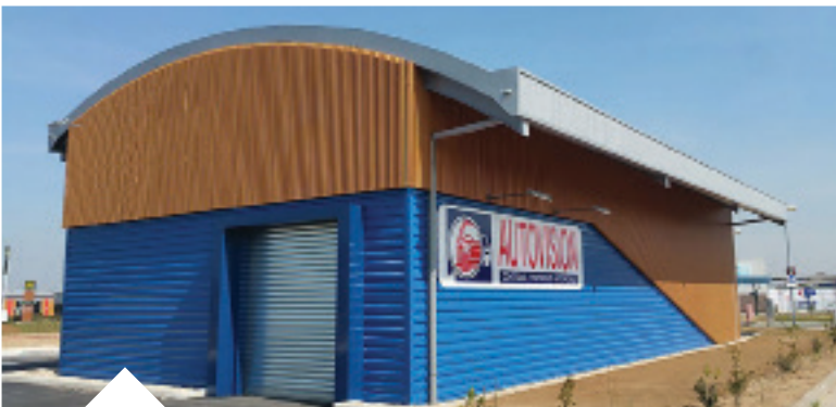
Autovision, FLINS-SUR-SEINE (78) Architect: Comodis Ingénierie | Installation: Soteba RSR
