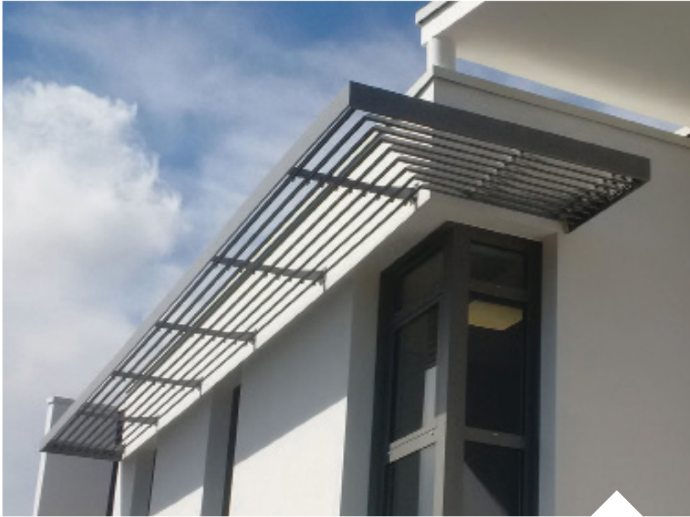
Public Notary Office, AIZENAY (85) Architect: Olivier DUGAST | Installation: Secom'Alu
