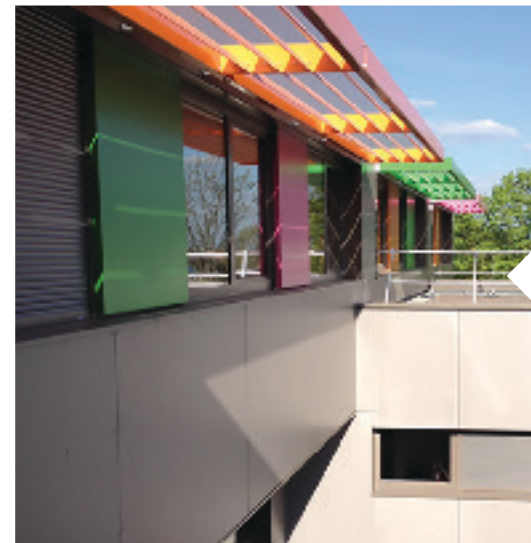
Middle School HOMBourg HAUT (57) Architect: Denu-Paradon | Installation: MTI
