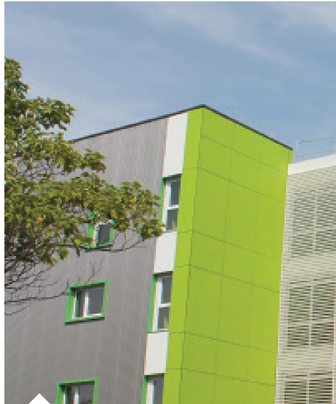
Residence CROUS, VILLETANEUSE (93) Architect: Sepra Architecture | Installation: Cougnaud et SMAC
