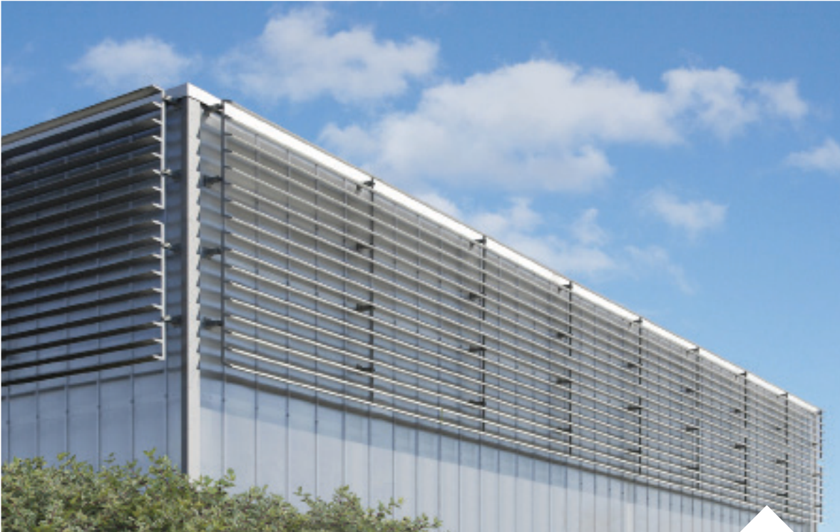
Gymnasium and martial arts dojo Jeanne d'Arc, REIMS (51) Architect: BLP architectes | Installation: SMAC
