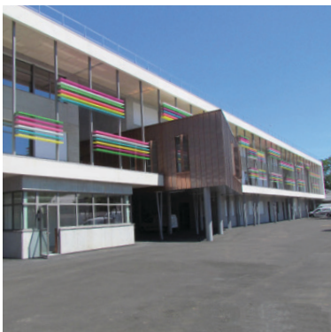
Middle School Montesquieu, ORLÉANS (45) Architect: Crea'ture Installation: Bernardi
