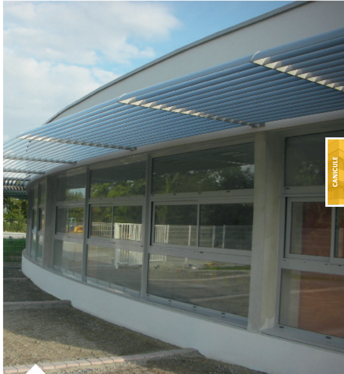
School, LE POIRÉ SUR VIE (85) Architect: Britton & Claude | Installation: Menuiserie Bertrand
