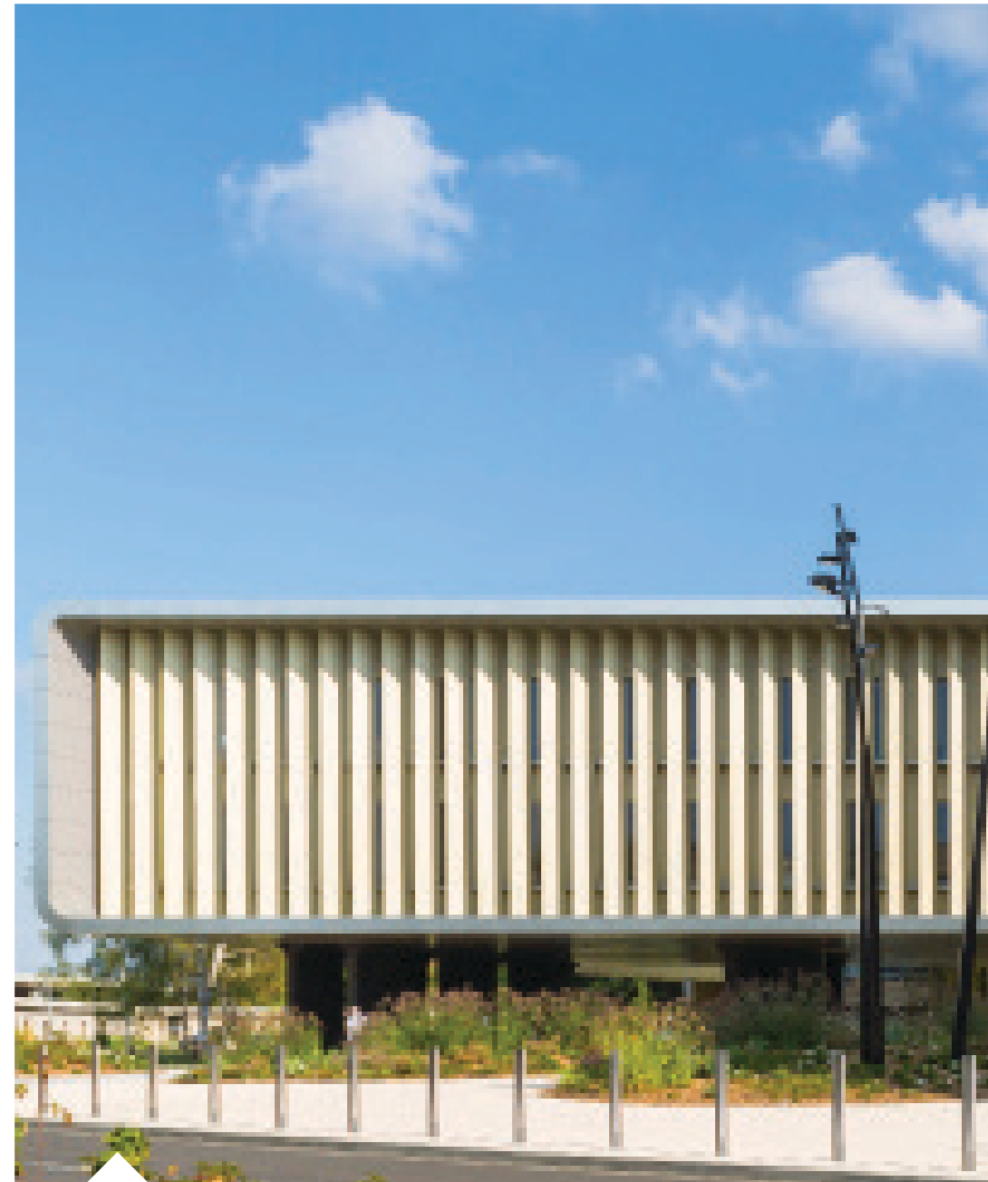
Hospital administration building CHU, POITIERS (86) Architect: Brenac & Gonzalez | Installation: BGN | Picture: Sergio Grazia
