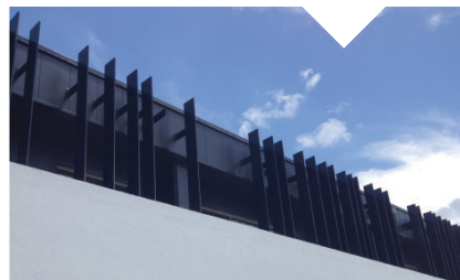
Campus IUT, AUXERRE (89) Architect: Geoffroy Zonca Installation: AD Metal
