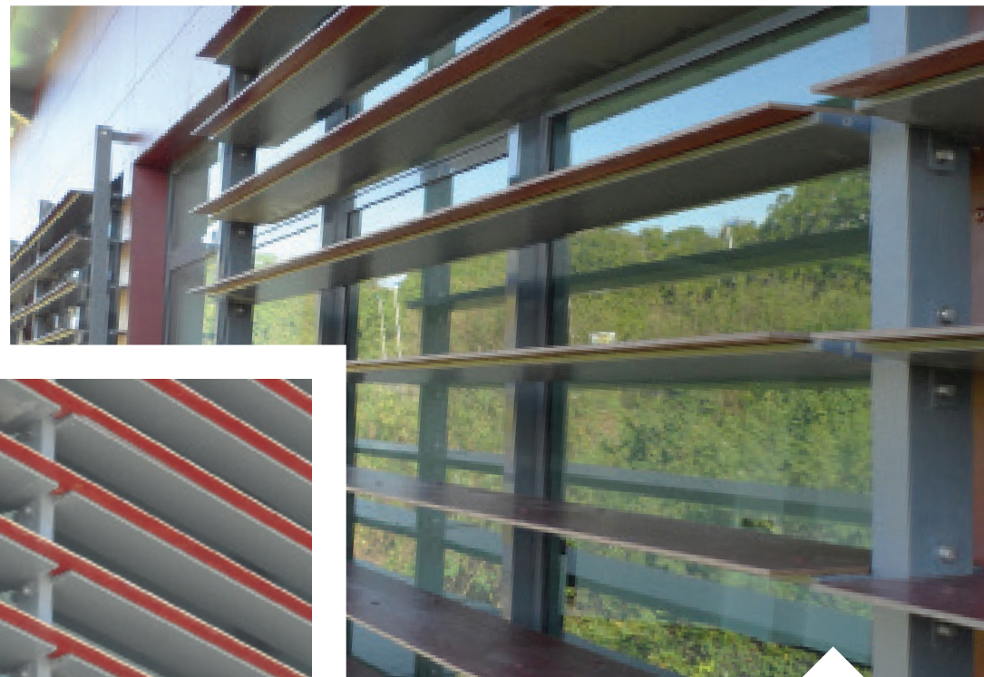
Activity hub Antillopôle, GUADELOUPE (97) Architect: Luc Martz & Associés | Installation: Métalu
