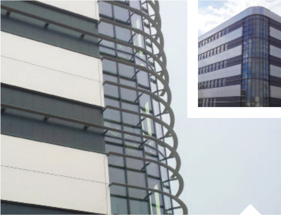
Headquarters RTE, LA CHAPELLE SUR ERDRE (44) Architect: Patriarche & Co | Installation: Girard Hervouet
