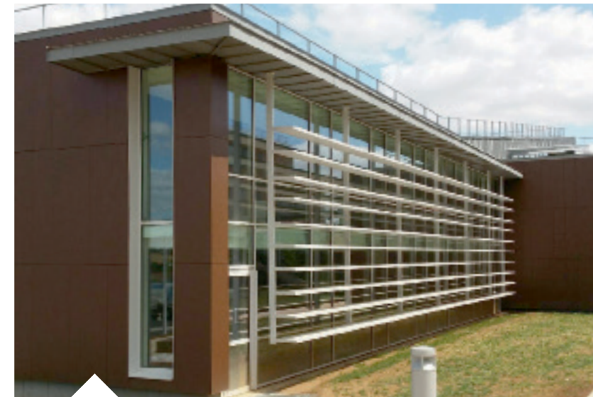
High School des Mauges, BEAUPRÉAU (49) Architect: Epicuria architectes | Installation: Ets David
