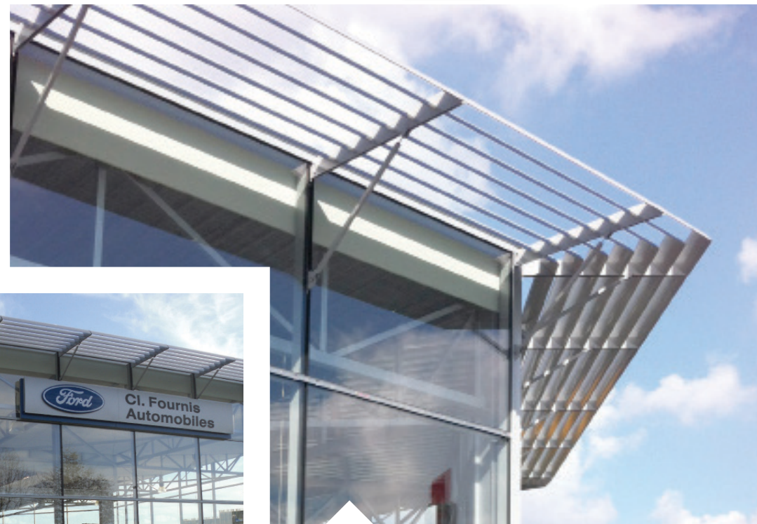
Car dealer shop Cl. Fournis Automobiles, HEROUVILLE SAINT CLAIR (14) Installation: Mestal
