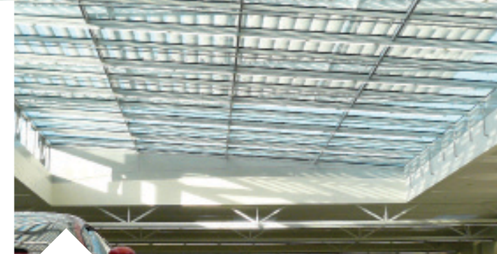
PSA, VÉLIZY (78) Architect: Atelier Ripaud
