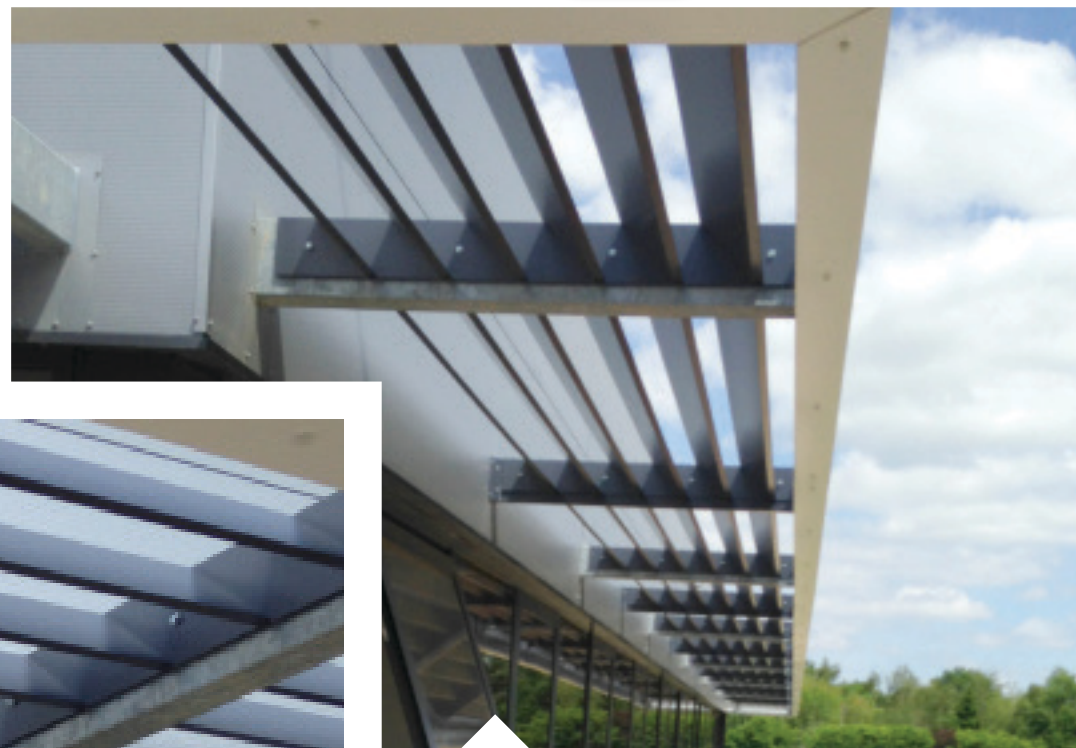
Centre viti-vinicole, BLANQUEFORT (33) Architect: Pascal Mollard | Installation: Face Aquitaine
