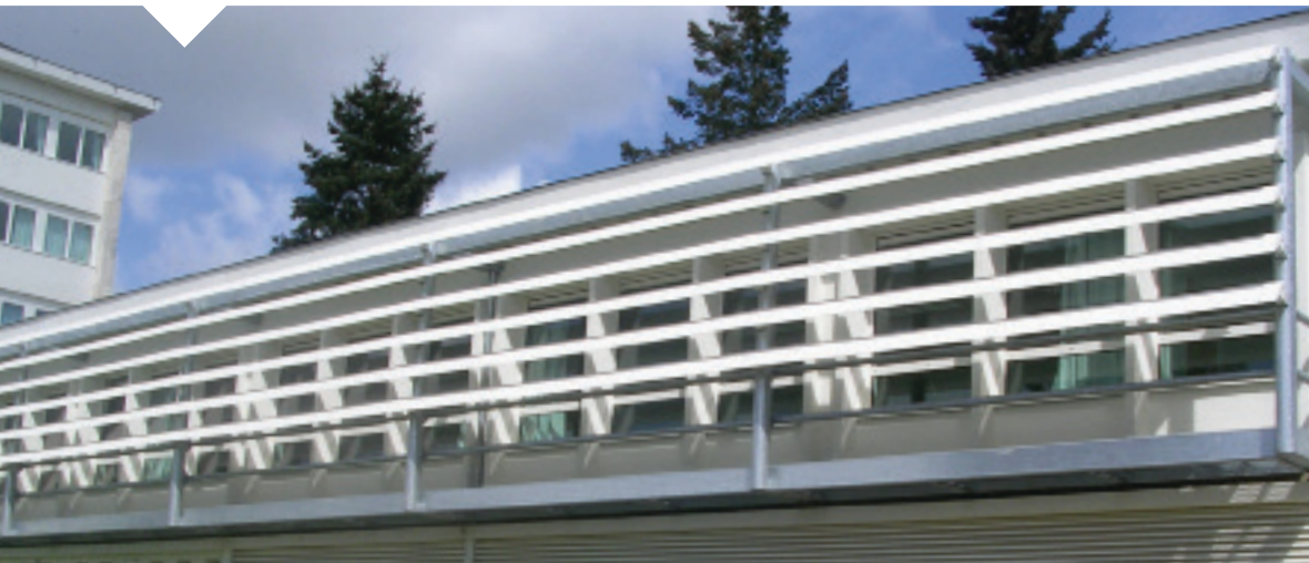
High School Chevrollier, ANGERS (49) Architect: Logerais & Associates | Installation: SAS Adrion
