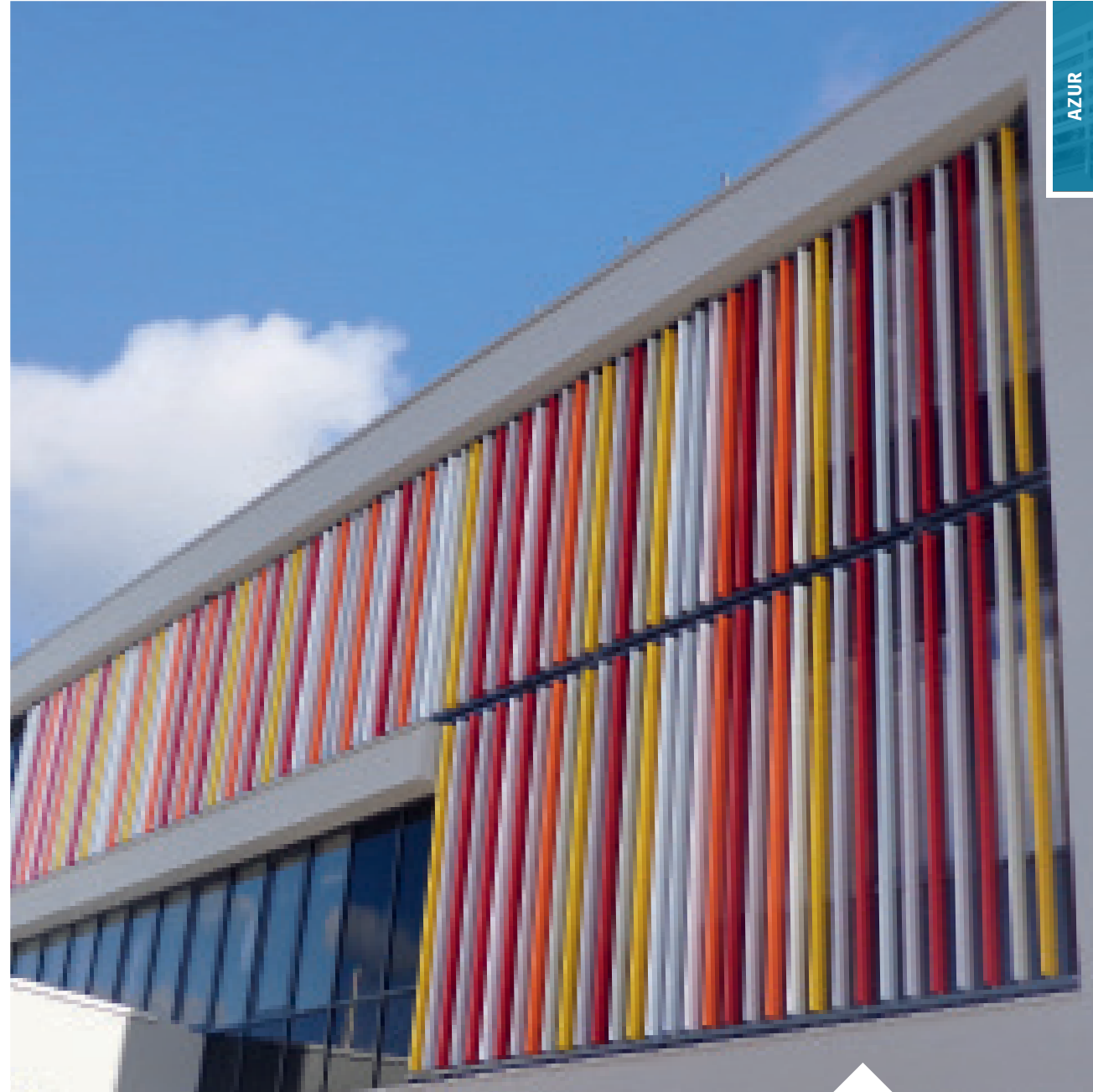
Middle School Milcendeau, CHALLANS (85) Architect: Linéa Architecte | Installation: Secom'Alu
