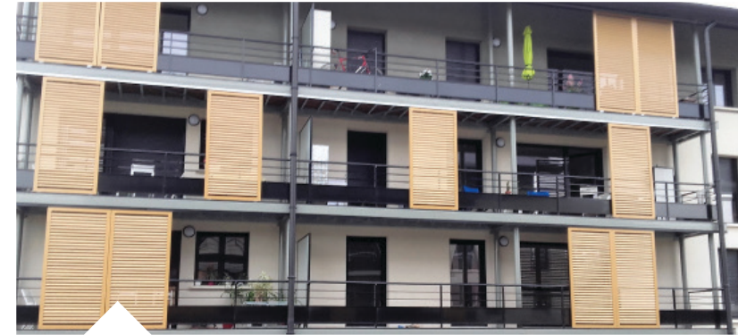
Multi-units building J.J. Rousseau, SOISSONS (02) Architect: Bellière-Manière Architectes | Installation: Aark
